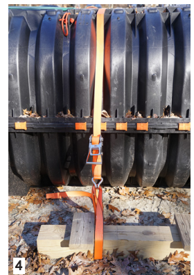
Position strap on beam.
