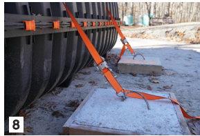
8 Connect strap to plate.
