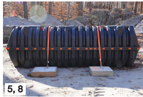
5, 8 Position straps on tank.
