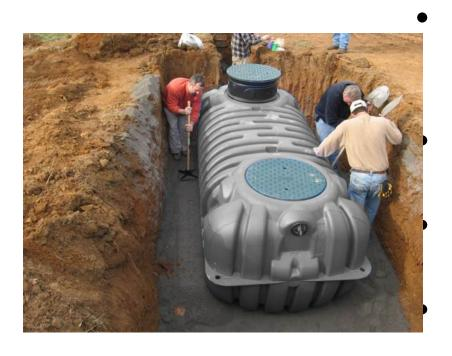
After getting material under the haunch of the tank, begin backfilling along sidewalls
