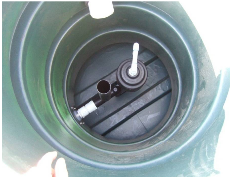
Figure 6. Dosing siphon - internal view
