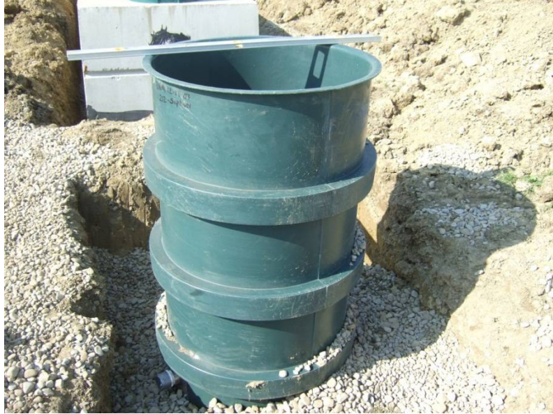
Figure 5. Dosing siphon - external view
